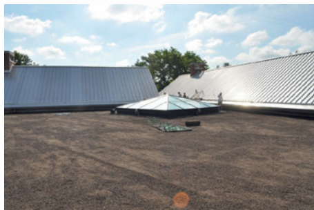
Roofing substrate prepared for installation
