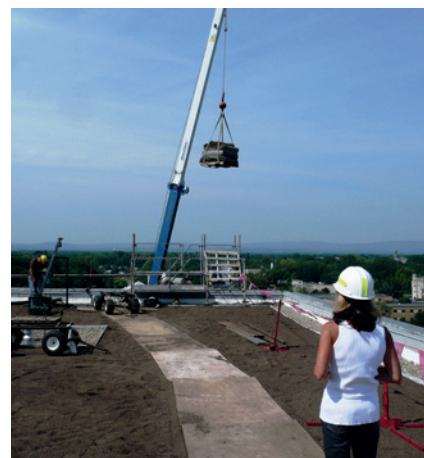
Plywood road to prevent soil compaction
